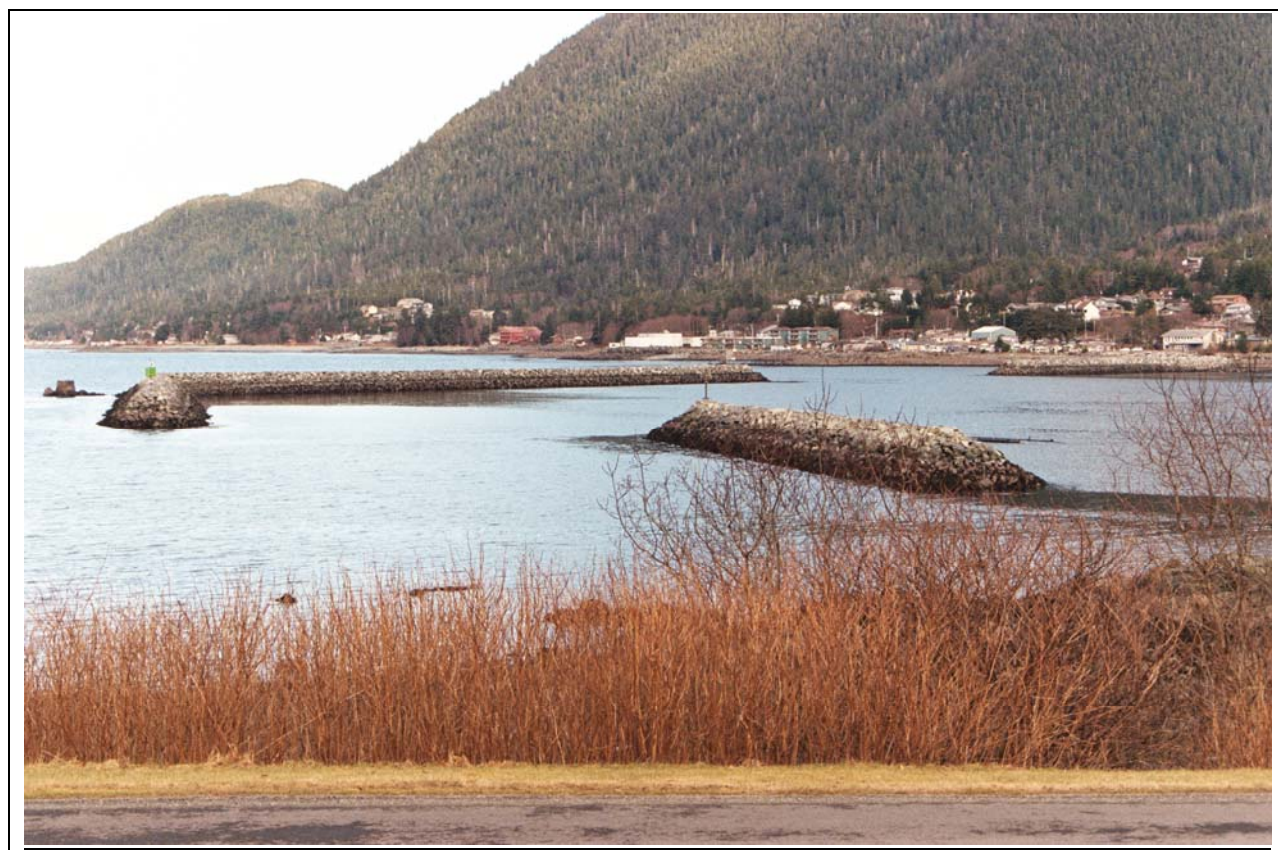
Figure 1: Breakwater ‘Gaps’ at the North End of Sitka Channel from Japonski Island
