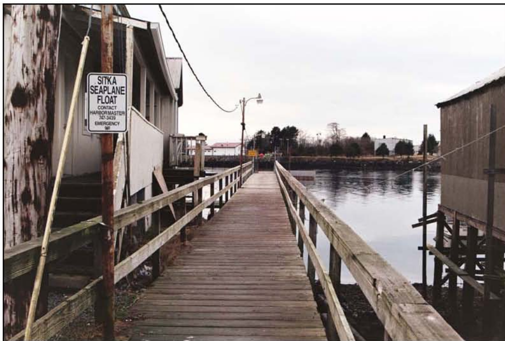
Figure 3: Access Walkway to Sitka Seaplane Float
