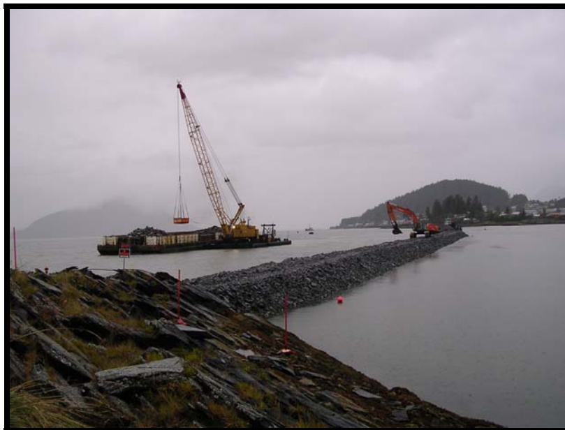
Photo 2. Skip box and crane off loading core material at Wrangell Harbor.
