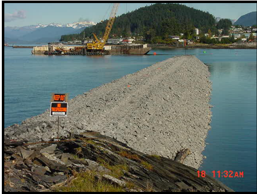
Photo 3. Core rock following shaping with excavator at Wrangell Harbor.
