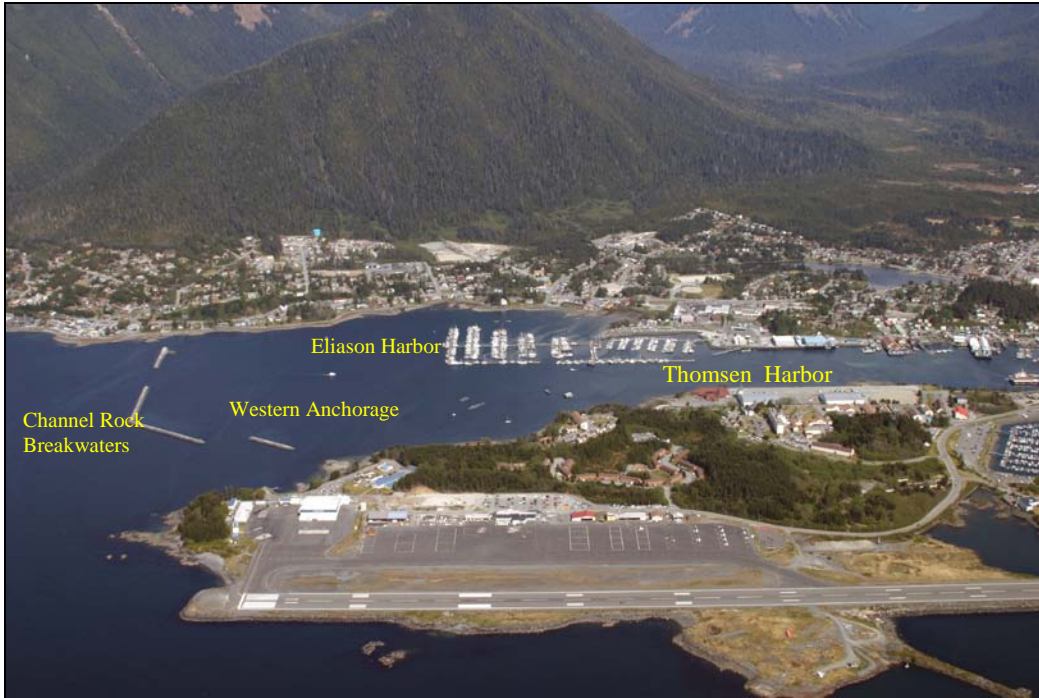
Figure 4. Sitka Harbors. Aerial photo from southwest, showing Thomsen Harbor, Eliason Harbor, Western Anchorage, and Channel Rock Breakwaters.
