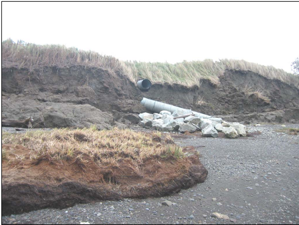
Figure 15: Disposal Area Berm at South Outfall, September 2005
