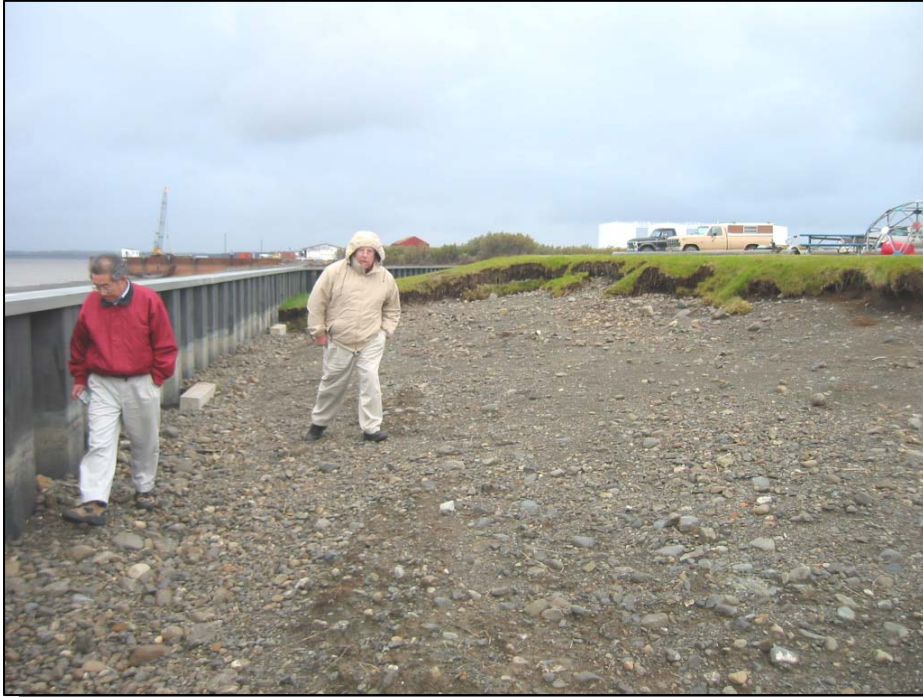
Figure 17: Seawall Erosion looking Eastward (September 2005) City Dock Side
