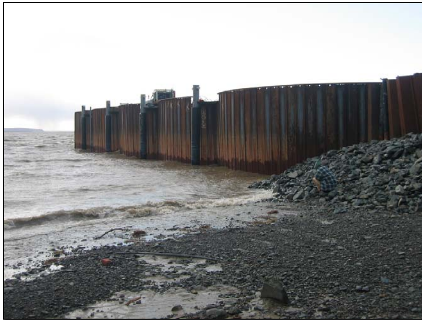
Figure 6: Dillingham Fuel Tank Farm Dock Protection
