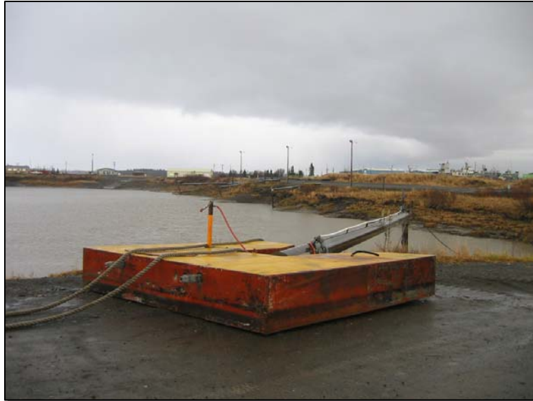
Figure 8: Float-to-Shore Connecting Swing Arms (on shore for winter) West End study area
