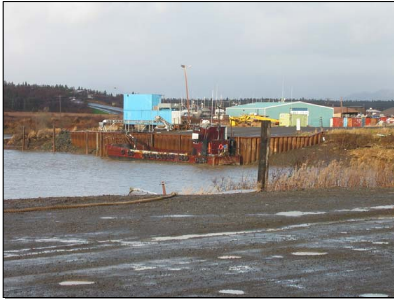
Figure 11: Harbor Bulkhead, North End of Dillingham Harbor West End study area
