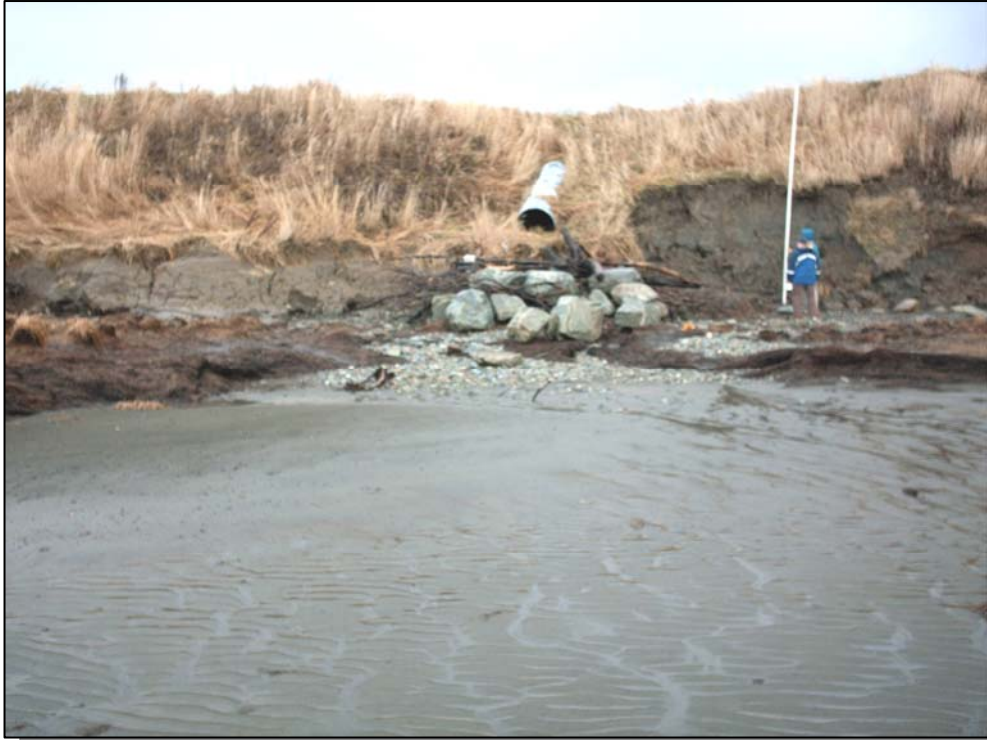
Figure 14: Disposal Area Berm at South Outfall, October 2004
