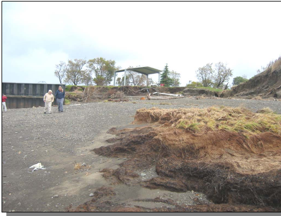
Figure 19: Erosion at Dillingham City Park looking North (September 2005)
