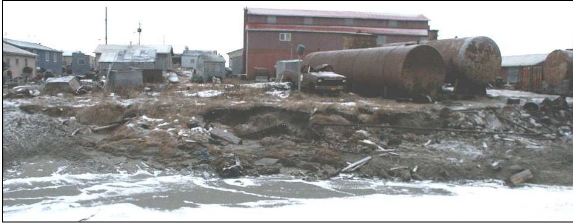
A store on Shishmaref and fuel oil provider with no protection.
