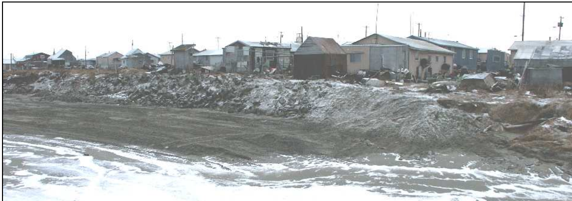
Significant numbers of residences have no erosion protection.
