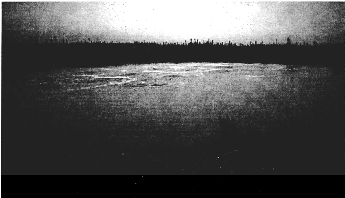
FIGURE J-7.—Aerated lagoon for wastewater treatment.
