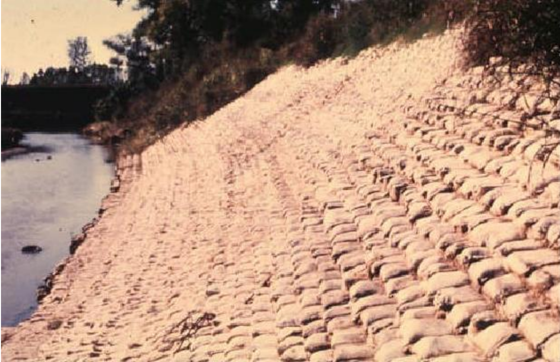
Figure 4.2: Typical soil-cement sack revetment.
