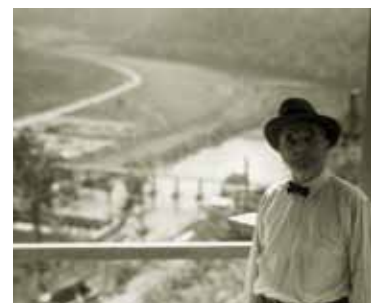
Construction overlook of the Norris Dam located in Anderson and Campbell Counties in Tennessee, c. mid-1930s.
