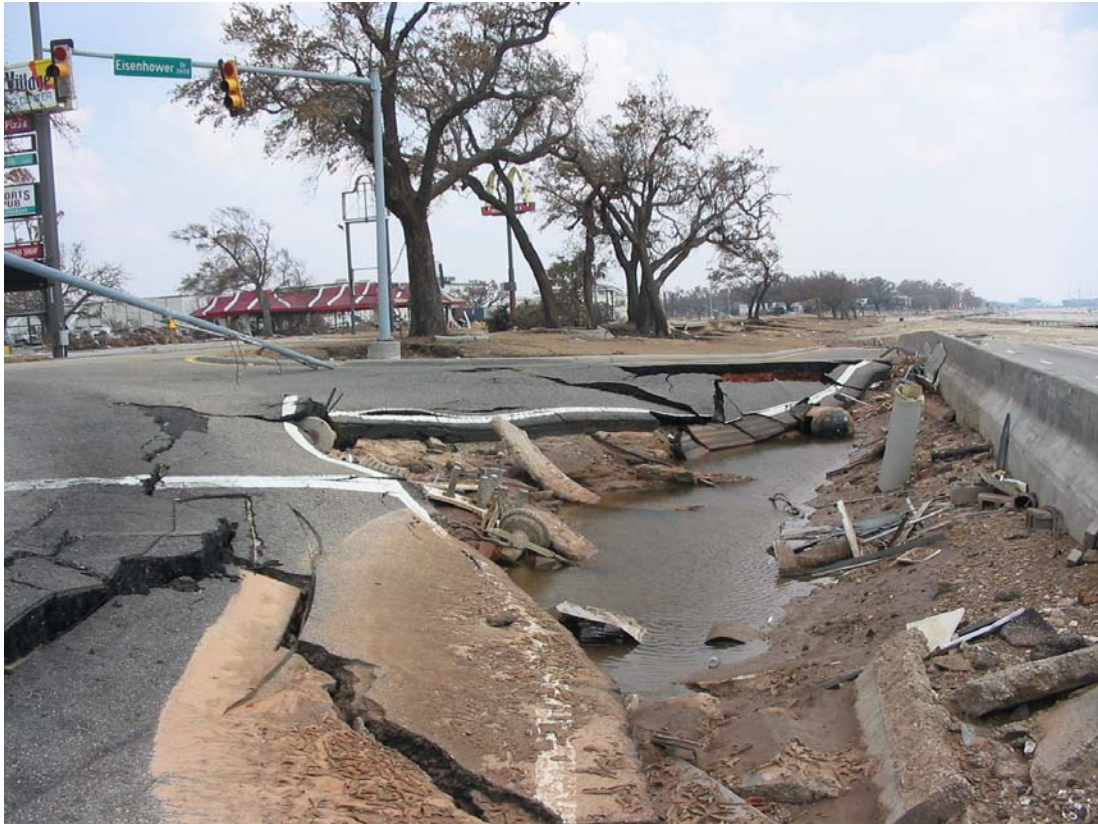
The damage from Hurricane Katrina made many roads around Keesler AFB impassible, even after workers had cleared debris from shattered houses and downed trees. In the distance, only a roof and vertical supports remain of a fast-food restaurant.
