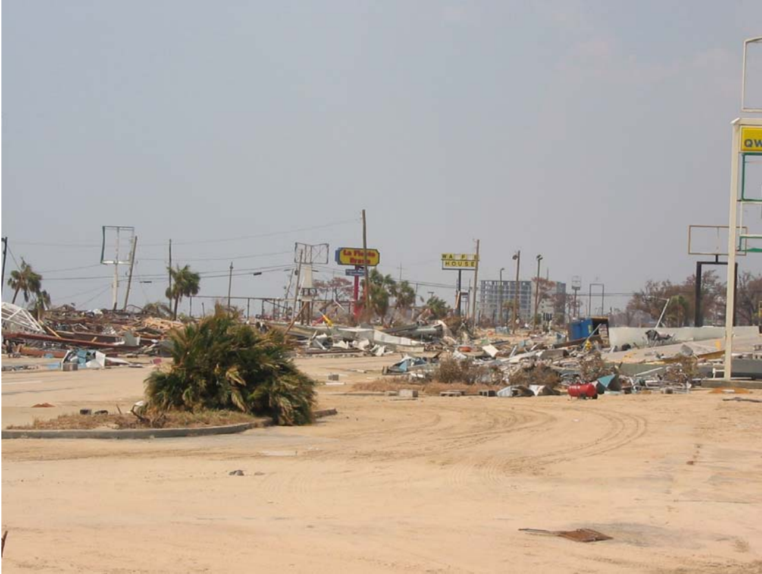
The storm surge from Hurricane Katrina devastated businesses along U.S. 90, the highway that passed through the coastal communities near Keesler AFB, Mississippi.
