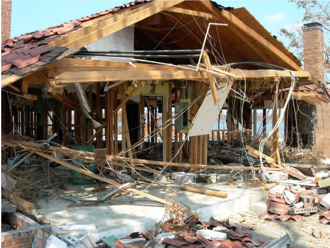
Military Family Housing units along the Back Bay of Biloxi were particularly hard hit by Hurricane Katrina’s storm surge, which raised water levels nearly 20 feet, flooding approximately half of Keesler AFB, Mississippi. The sites with the lowest elevations above sea level were abandoned as Keesler planned to rebuild its housing units (photo by Capt Brady Smith).
