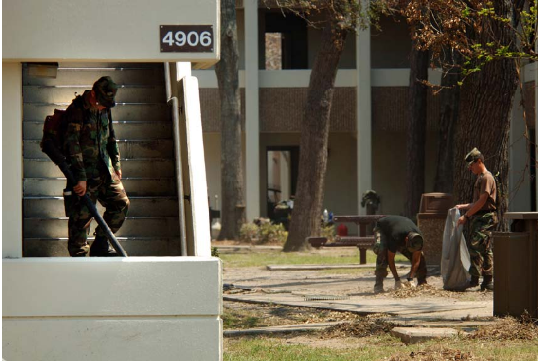
With training operations suspended at Keesler and students evacuated, 400 Airmen stayed behind to clear the base of debris left in the wake of Hurricane Katrina's destructive path (USAF photo by MSgt Efrain Gonzalez).
