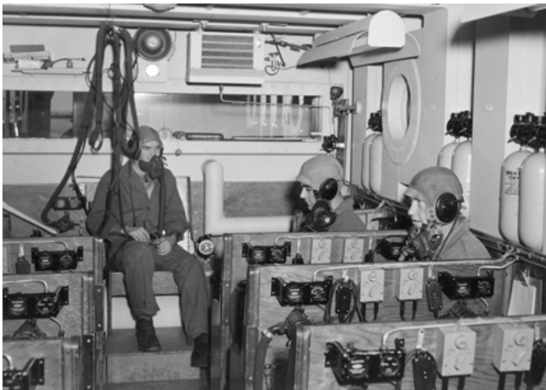
At Vance AFB, Oklahoma, pilot trainees use the altitude chamber to simulate flying at high altitudes.
