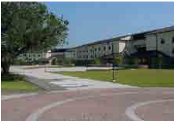
This new student dormitory at Keesler AFB was built to the new standards adopted in the Dormitory Master Plan.
