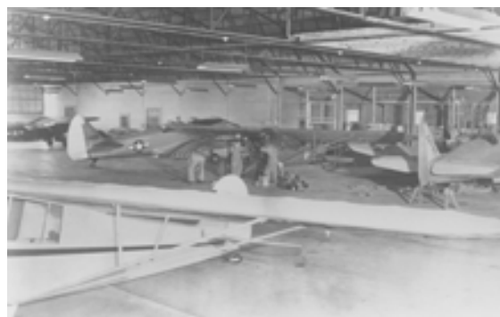
Aircraft mechanics work on L-4 aircraft at Denton Texas, in October 1943.
