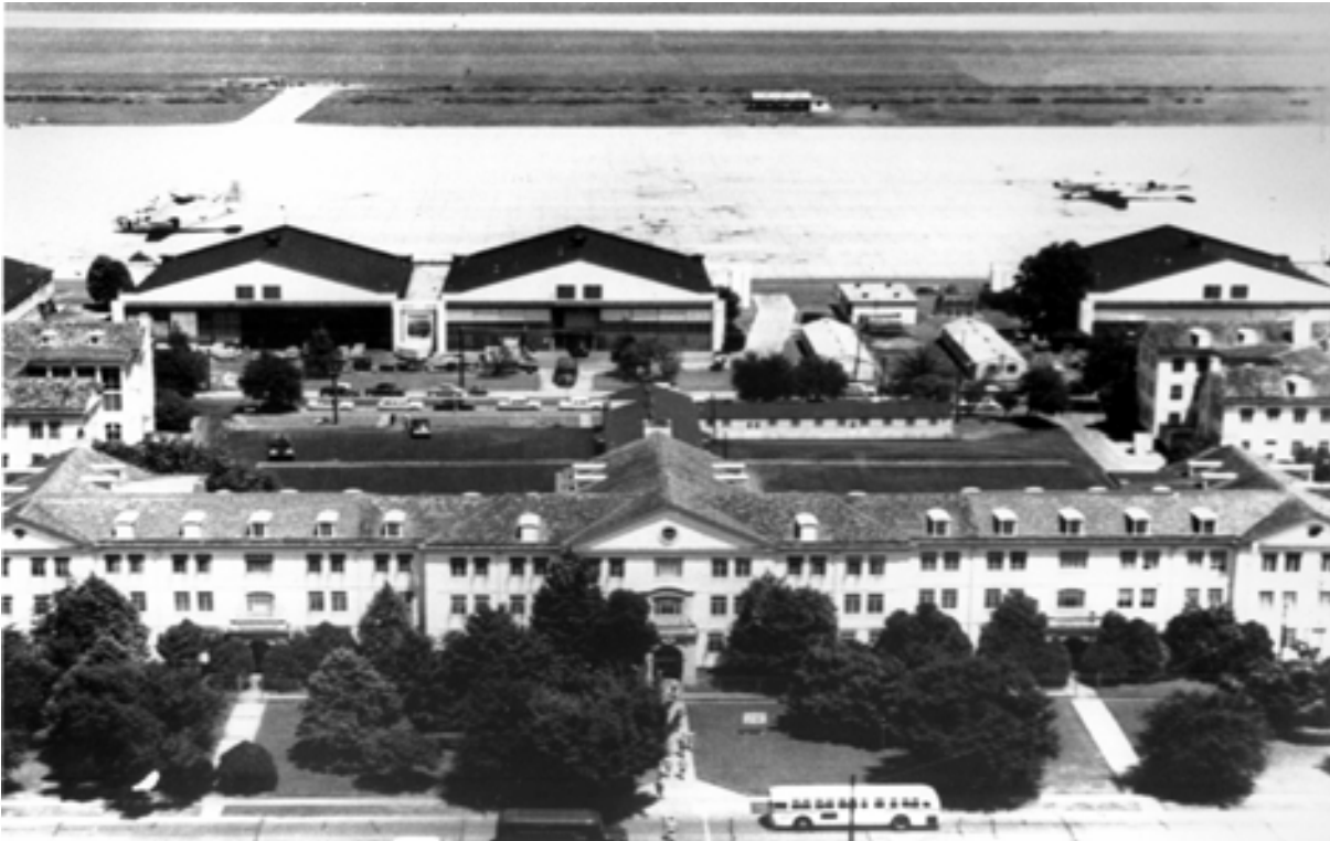
In February 1947 Training Command moved its headquarters from downtown Fort Worth, Texas, to Barksdale Field in northwestern Louisiana. In the foreground of the above photo, is the new headquarters building.
