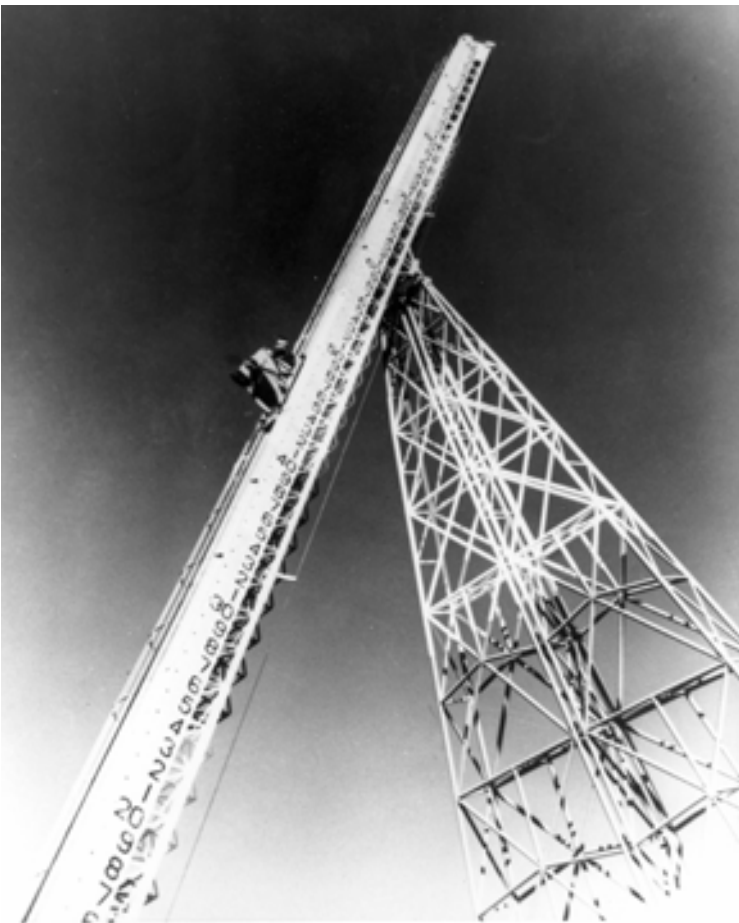
The TE-105A Ejection Seat Trainer, more commonly known as the "Boom Bucket," was erected at Williams AFB, Arizona, in 1949. This trainer, the only one of its kind in the Air Force, simulated ejection from a jet aircraft. By the last ride on 30 July 1974, a total of 18,187 students had used the trainer.
