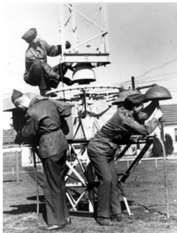
These communications students at Scott AFB, Illinois, are setting up a radio range station antenna.
