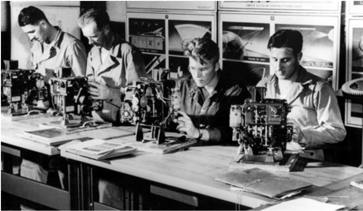
The bombsight was the key to successful missions. Here, Lowry students inspect and adjust Sperry bombsights.
