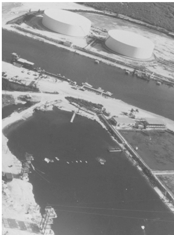
Shown are the remains of the Turkey Point water survival training complex located near Homestead AFB after Hurricane Andrew struck the Florida coast. As an interim measure, the Air Force relocated the Water Survival School to Tyndall AFB on Florida's gulf coast.
