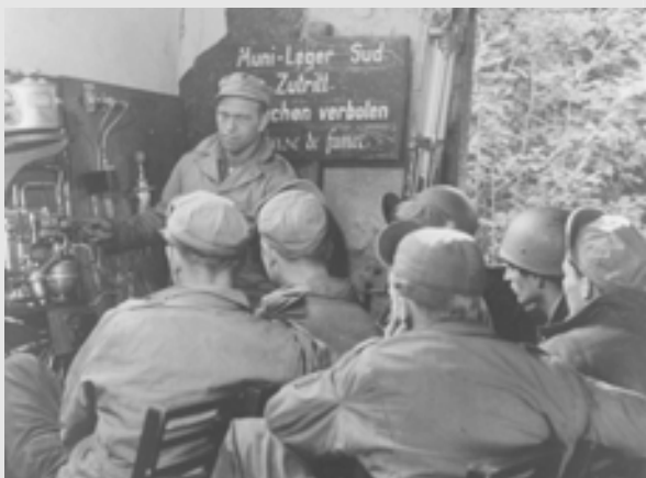
A mobile training unit instructor turns a bombed building formerly used by the German Air Force into a classroom for P-47 aircraft mechanics.
