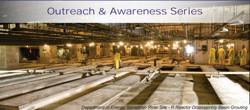
Department of Energy, Savannah River Site - R Reactor Disassembly Basin Grouting
