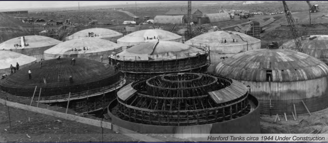
Hanford Tanks circa 1944 Under Construction
