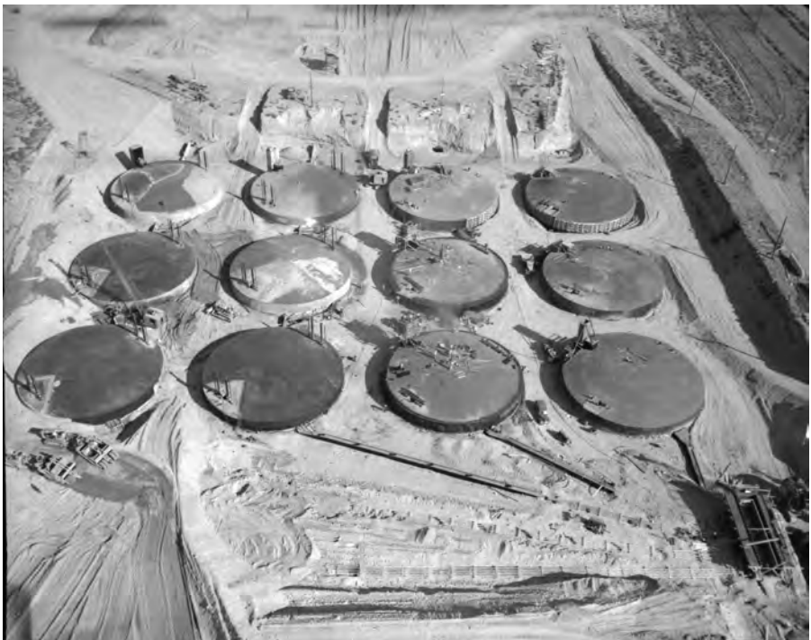
Hanford Tanks circa 1944 Under Construction
