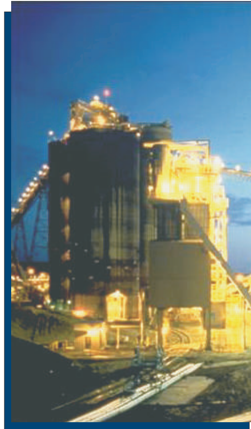
LIQUID PHASE METHANOL PROJECT
