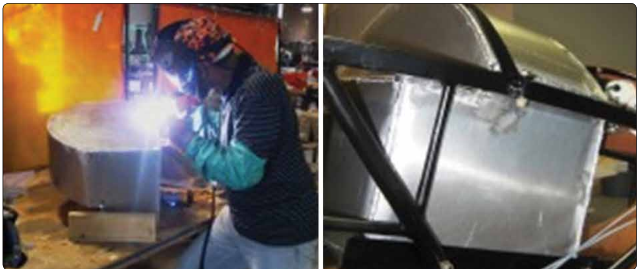
Figure 14-91. A rigid removable fuel tank with welded seams is repaired by welding.
