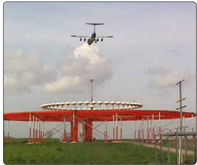
Figure 11-119. A VOR with DME ground station.
