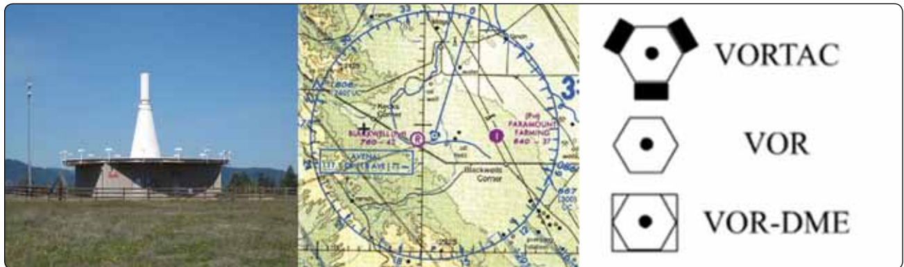
Figure 11-95. A VOR ground station.
