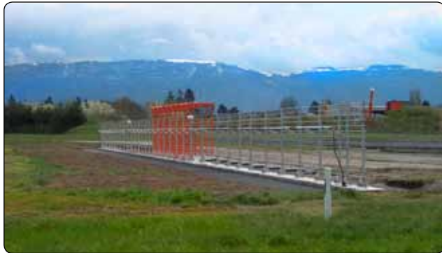
Figure 11-111. An ILS localizer antenna.
