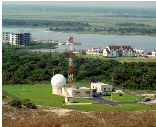
Figure 8-2. PDL Ground Station
