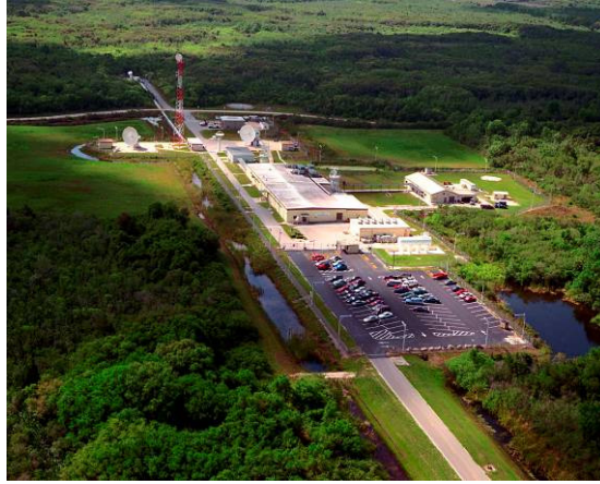
Figure 8-1. MILA Ground Station
