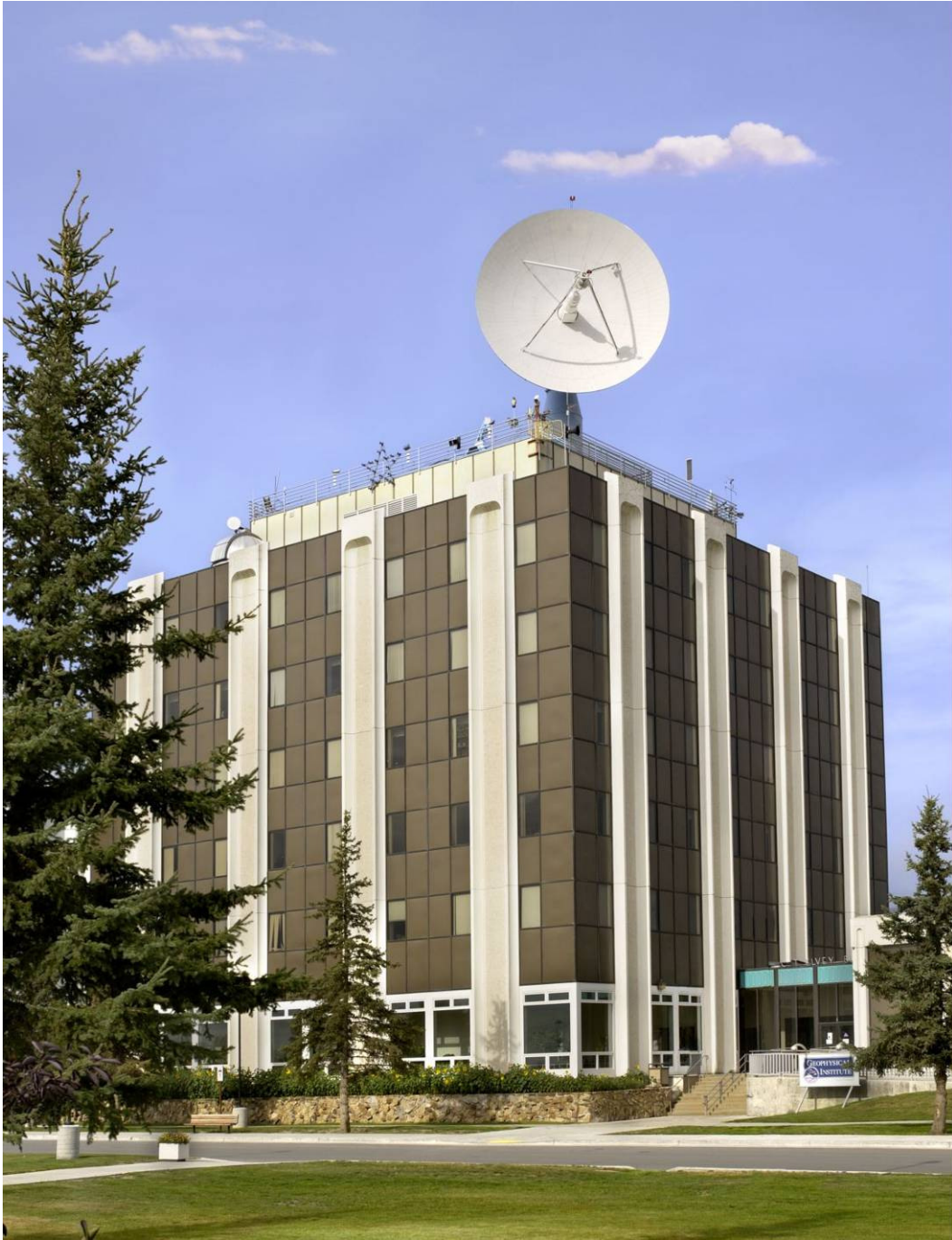
Figure 7-1. ASF 10-meter Antenna
