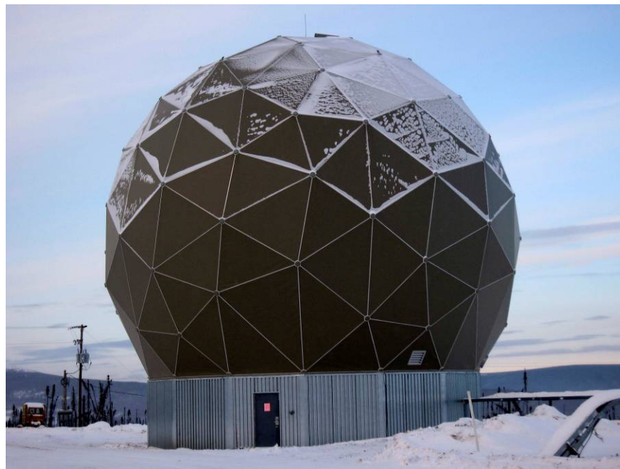
Figure 6-2. PF2 Antenna Radome
