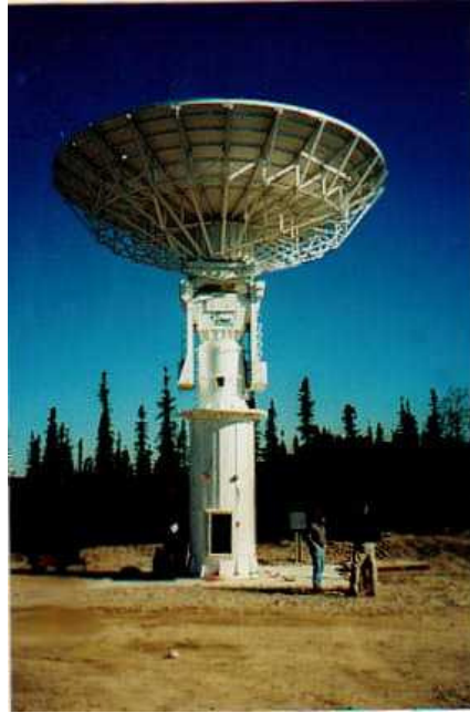
Figure 6-2a. PF2 Antenna Before Radome Installation
