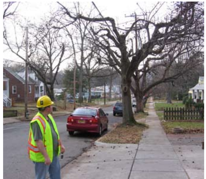
Conflicts between large trees and utility lines have a great impact on reliable power transmission and long-term tree health.
