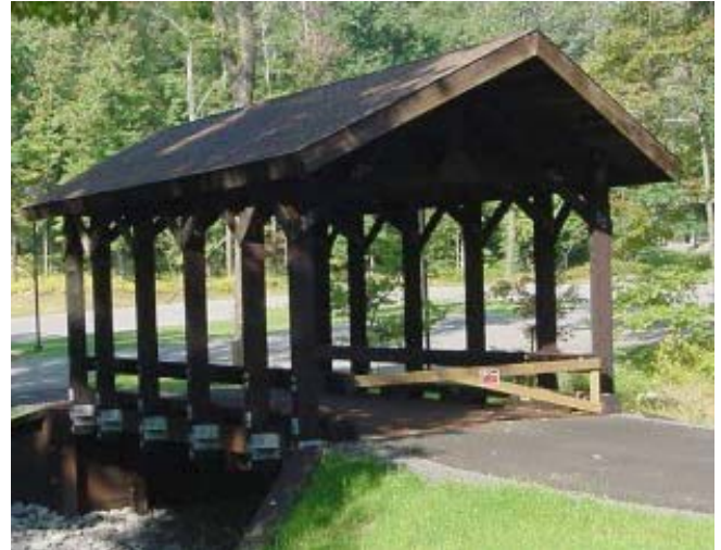
Parallam PSL was used in the recently constructed bridge at the entrance to the West Virginia University Division of Forestry's Natural Resource Center near Morgantown.
