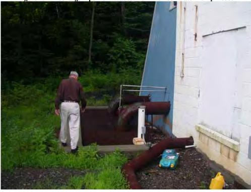
Figure 15 – Discharge Pipe from Wadesville Mine Pool Water Pump House
