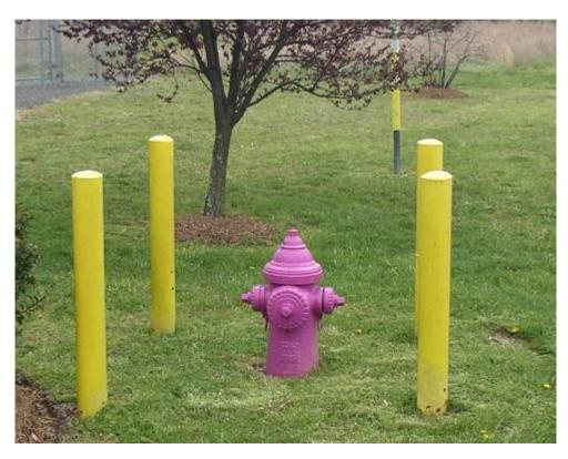
Figure 4 – Fire Hydrant Conveying Reclaimed Water (Source: Veil 2007)
