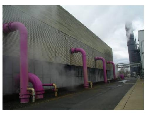
Figure 6 – Reclaimed Water Lines and Cooling Tower (Source: Veil 2007)
