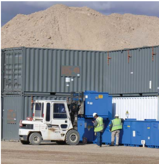
Area 5 Radioactive Waste Management Site personnel stack approved waste containers in a low-level waste disposal cell.
