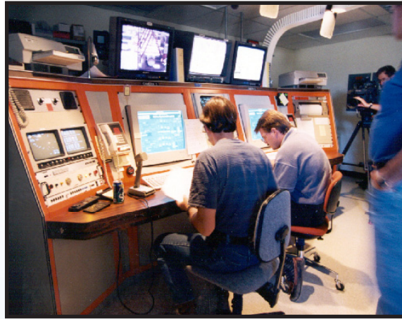
Tests are monitored from the Command, Control and Data Acquisition System building.
