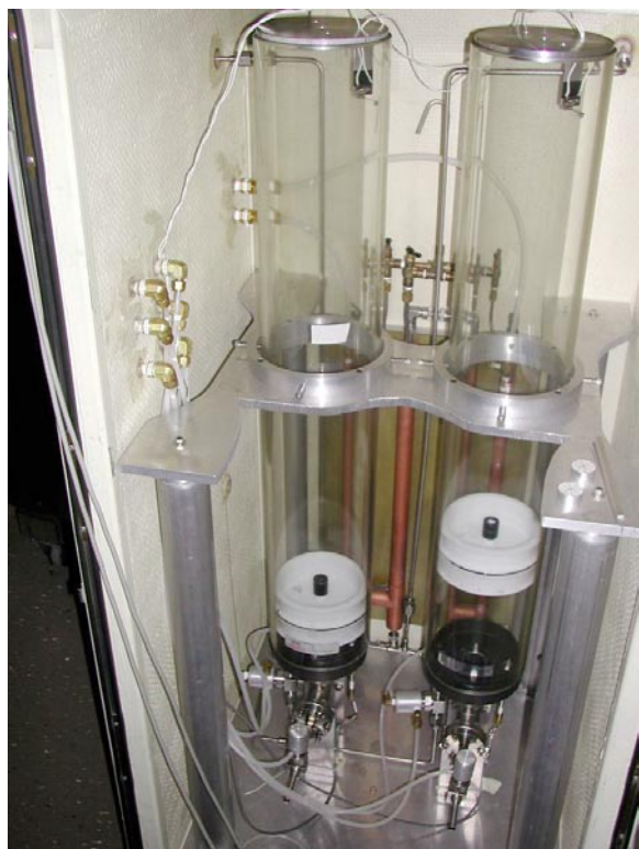
FIGURE 4. Photograph of dry gas collection facility for NIST gravimetric hygrometer.
