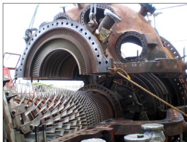
FIGURE 2. Removal of SGT-900 turbine casing
