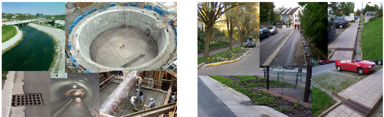
Replacing gray, centralized and monofunctional wastewater and stormwater infrastructure (left) with green, decentralized and multifunctional infrastructure (right) improves urban ecohydrology, ecology, and overall environmental quality.
