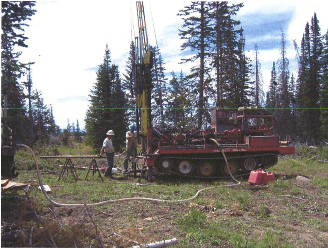
Boring B-101 Drill Rig Setup
