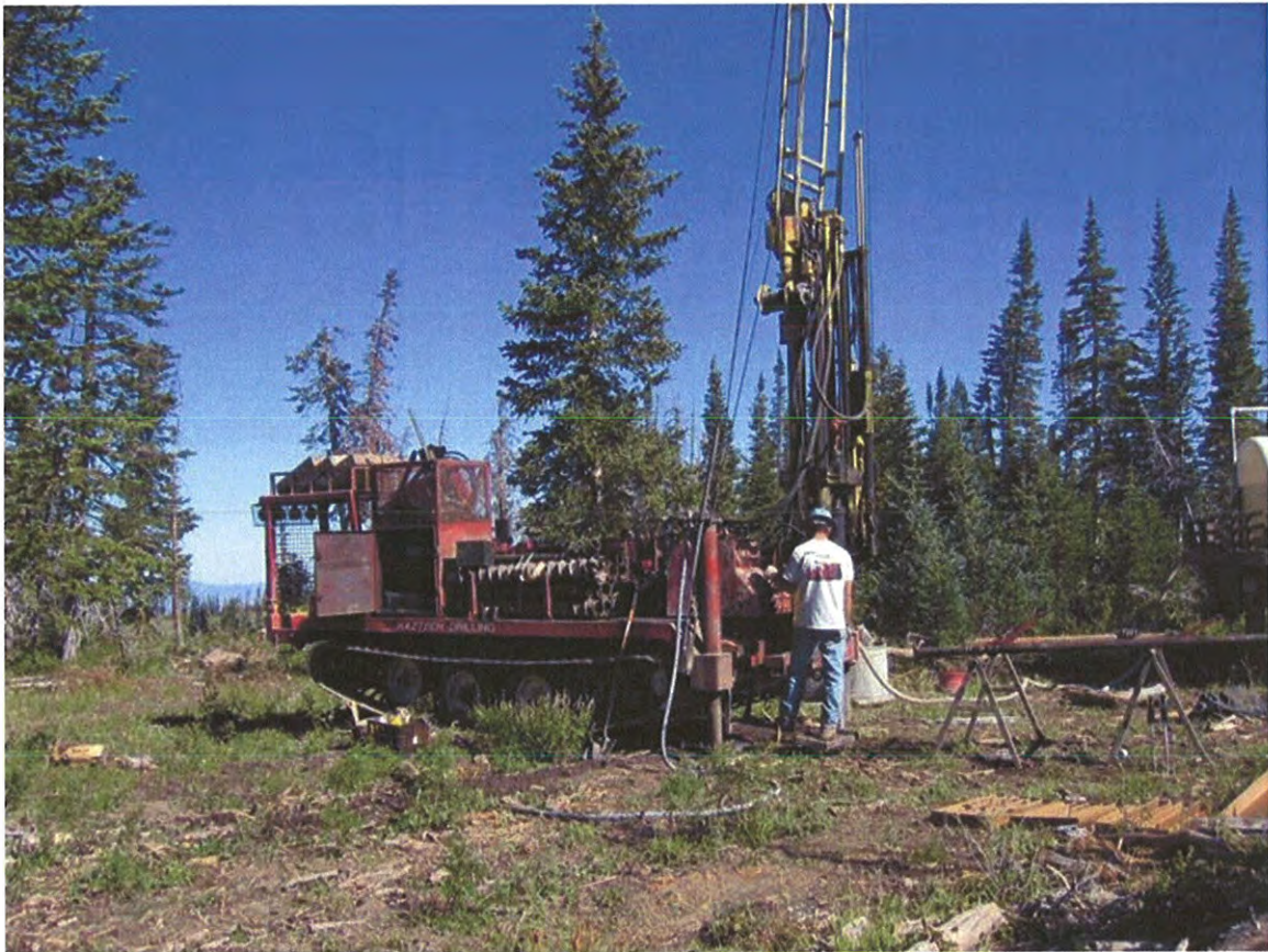
Boring B-102 Drill Rig Setup
