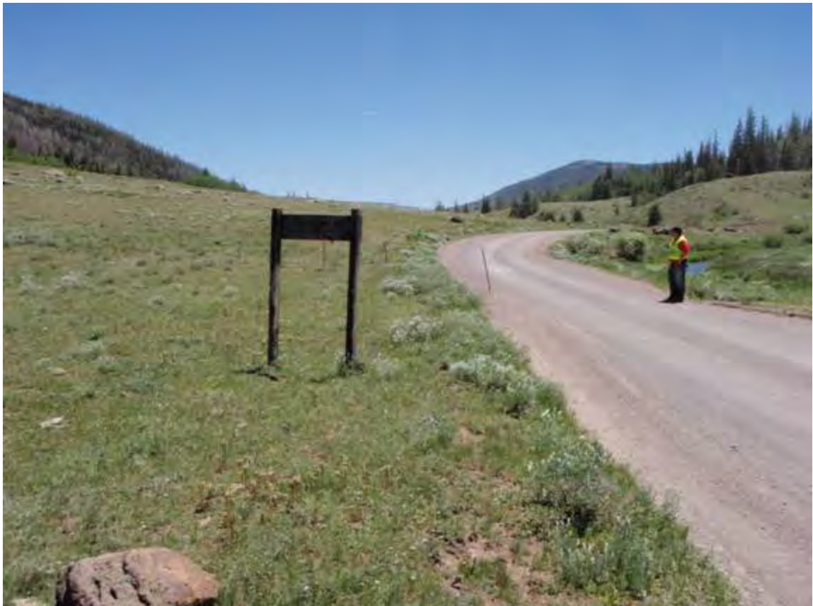
Station 79+00, Back On Line (BOL)
