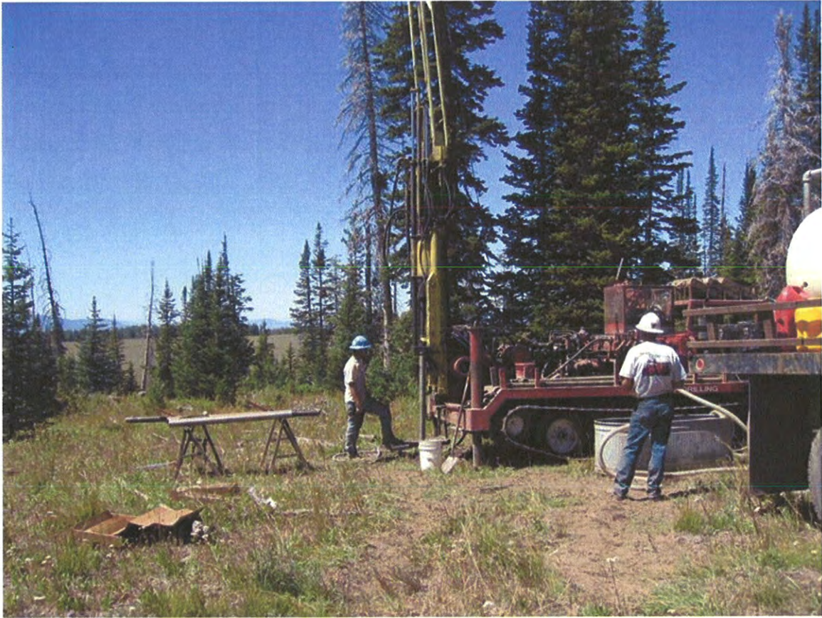
Boring B-104 Drill Rig Setup
