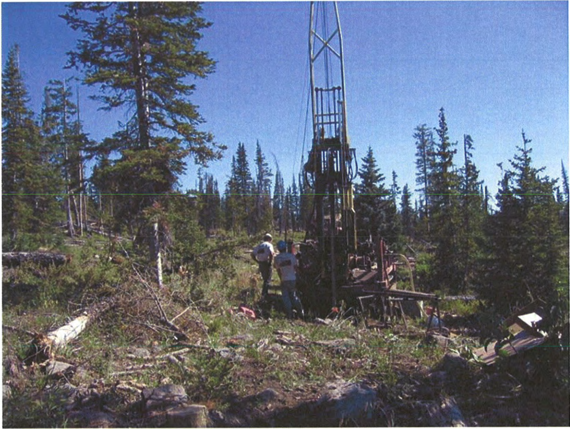
Boring B-105 Drill Rig Setup
