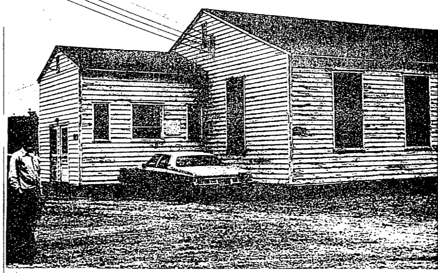
(F) EXTERIOR OF BUILDING LOOKING SOUTH EAST.
