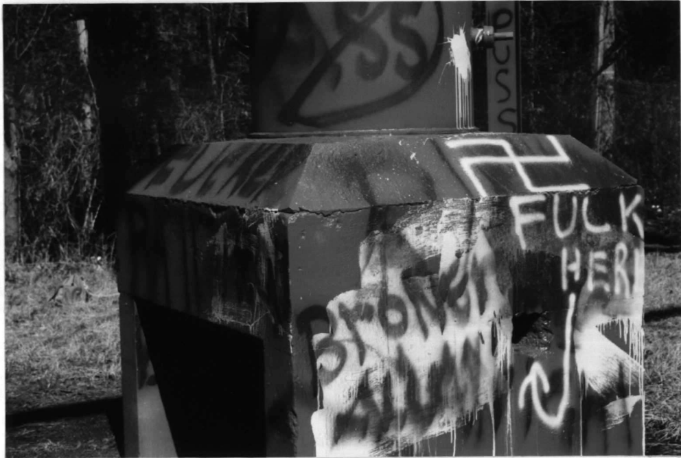
PHOTO NO. 17 STC-1070
