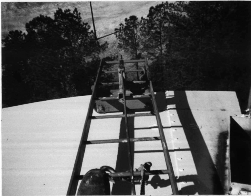
PHOTO NO. 1 STC-1070
