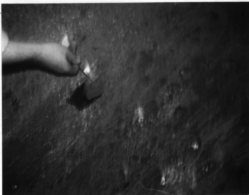
PHOTO NO. 19 STC-1070
