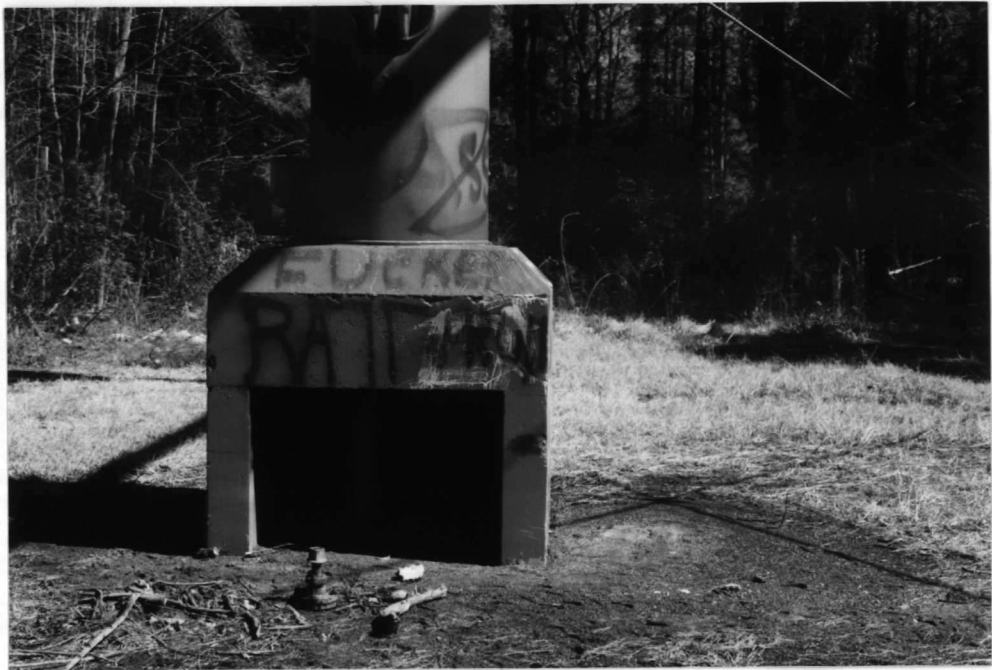
PHOTO NO. 7 STC-1070
