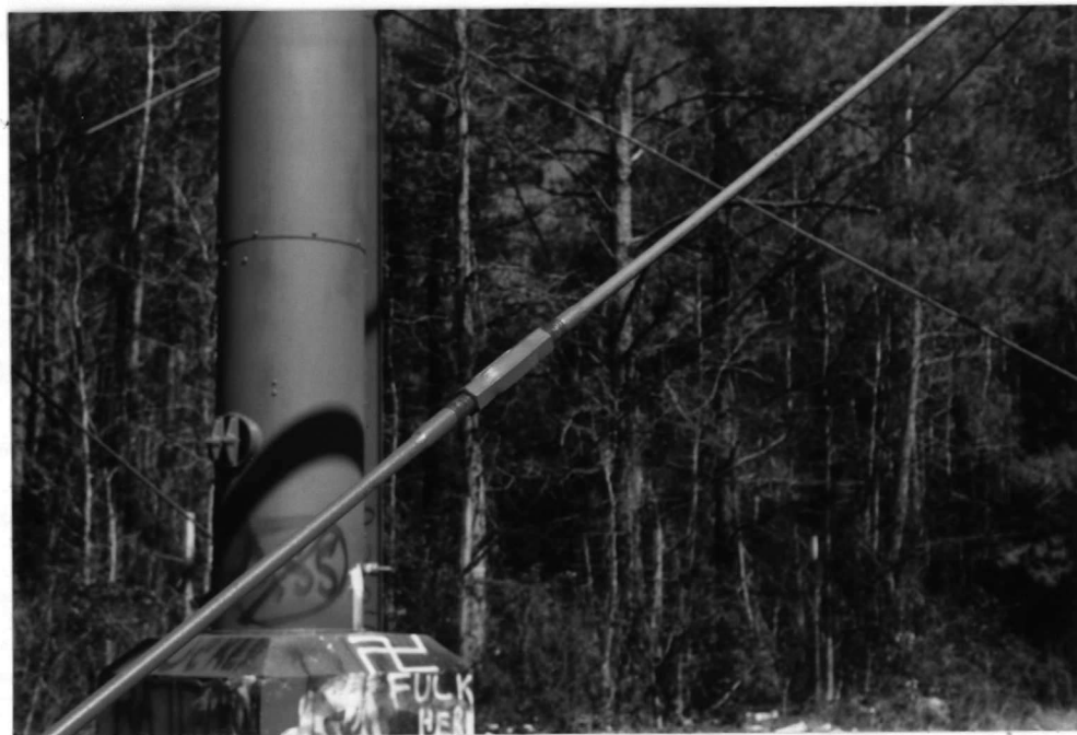
PHOTO NO. 12 STC-1070
