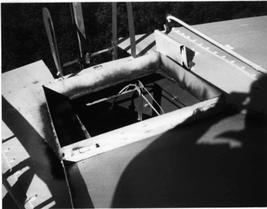
PHOTO NO. 2 STC-1070
