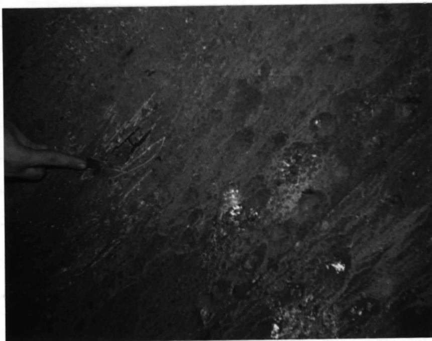
PHOTO NO. 20 STC-1070
