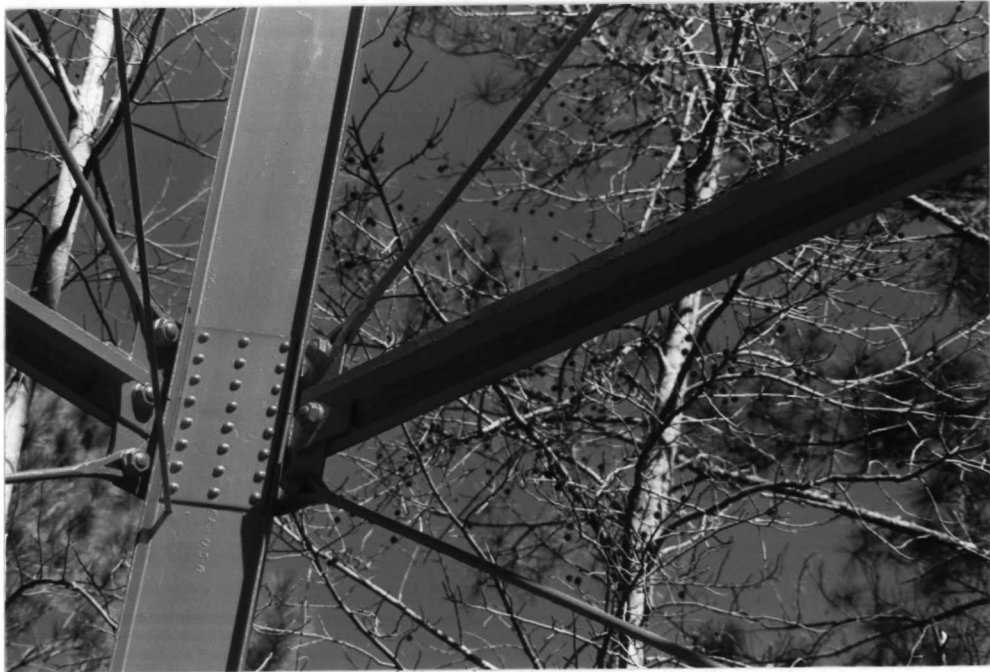
PHOTO NO. 16 STC-1070
