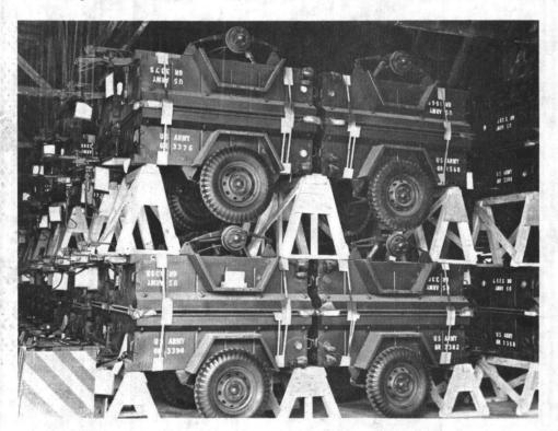
Figure 5-24. Wood stands for stacking vehicles in storage.
