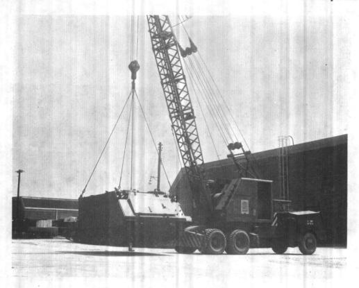
Figure 5-39. Truck-mounted crane.
