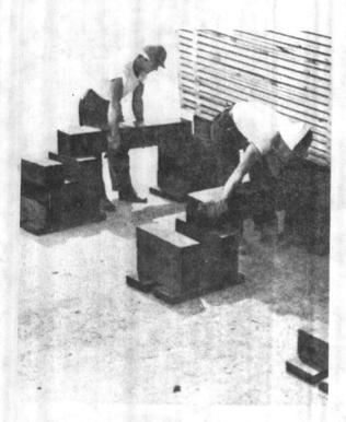
Figure 5–10. Application of the portable lumber foundation.
