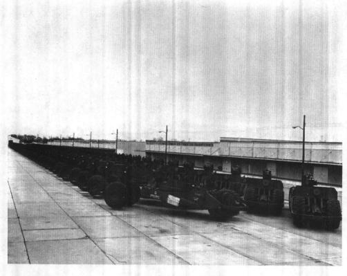
Figure 5-43. Modified back-to-back (herringbone) storage pattern. (Note: This pattern allows items to be driven or maneuvered directly into their locations with minimal handling.)
