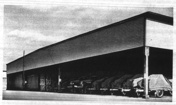
Figure 2-9. Shed storage showing the utilization of tarpaulins as end walls.
