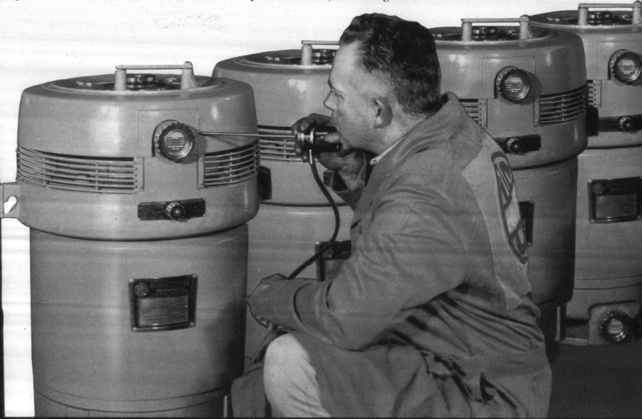
Maximum allowable vibration .00084"
