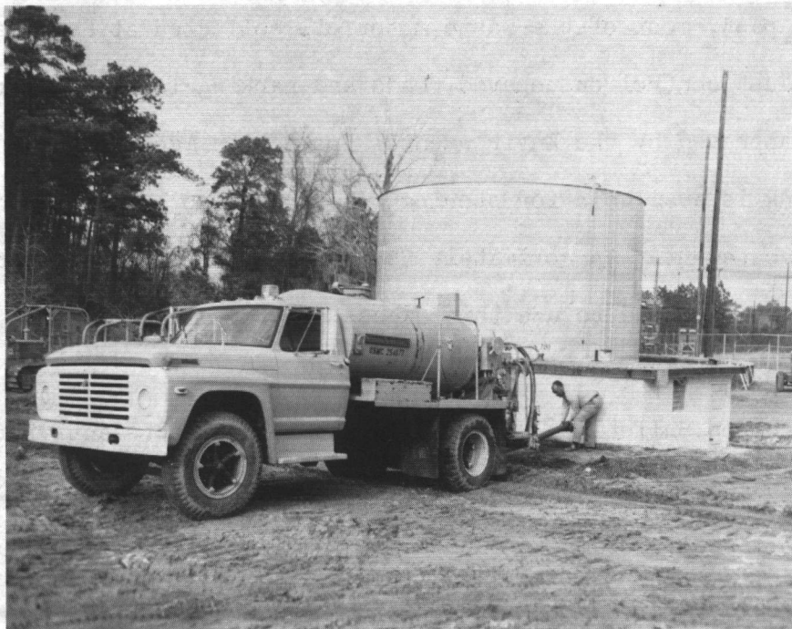
WASTE OIL COLLECTION TRUCK EMPTYING INTO THE 272,000-GALLON STORAGE TANK
