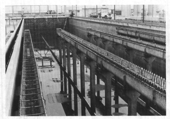
Dewatered sedimentation basin (Note inlet baffle at far end and traveling bridge above baffle)
