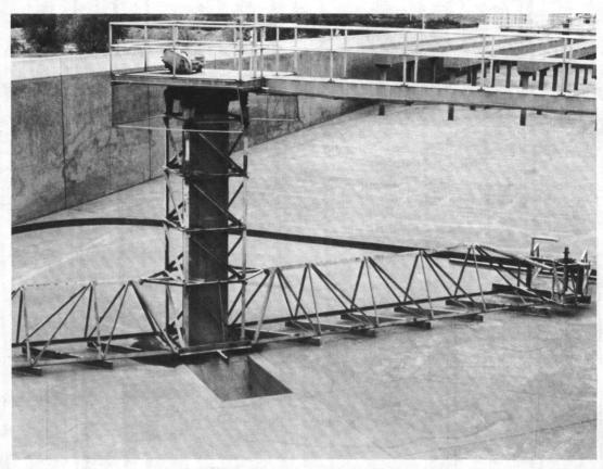
NOTE: Sludge sump is hole in middle.
