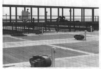
Traveling bridge (top) sludge removal system (Note covered flocculators in foreground)
