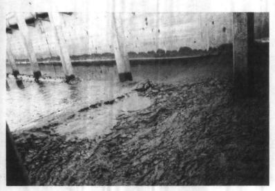
Fig. 5.6 Sludge buildup in bottom of sedimentation basin
