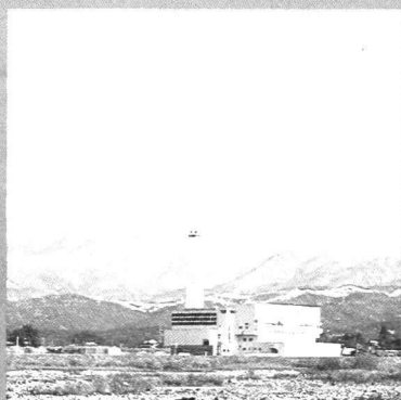
Toyama City (660TPD : 220TPD × 3 Units)
