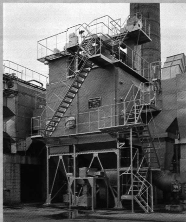
Heat Recovery Boiler
