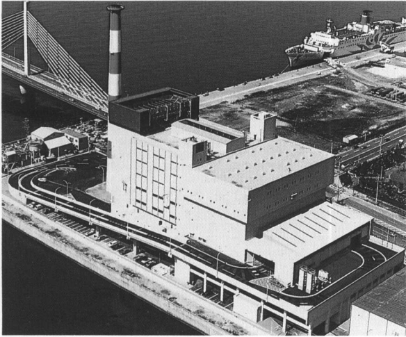
Osaka City Plant, 800 tpd
