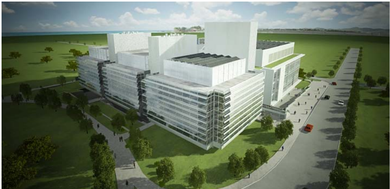
View of PNRC showing Phase I (to the left) & Phase II (to the right). Note the green roof ledges over PNRC II
