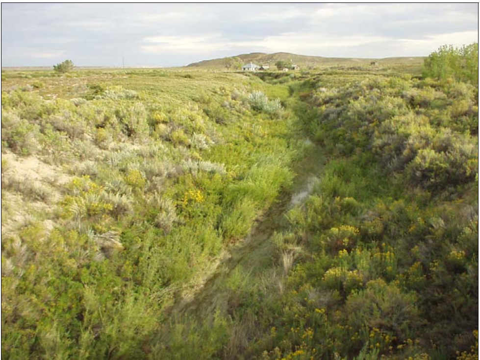
Figure 10. Muddy Creek Station G52 Upstream (above) and Downstream (below)
