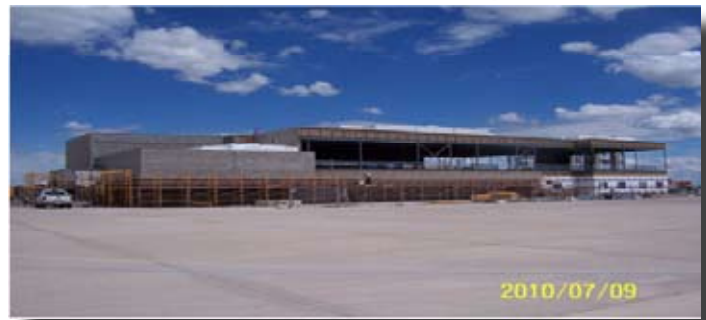
West side, Squadron Operations Facility, 35% complete
