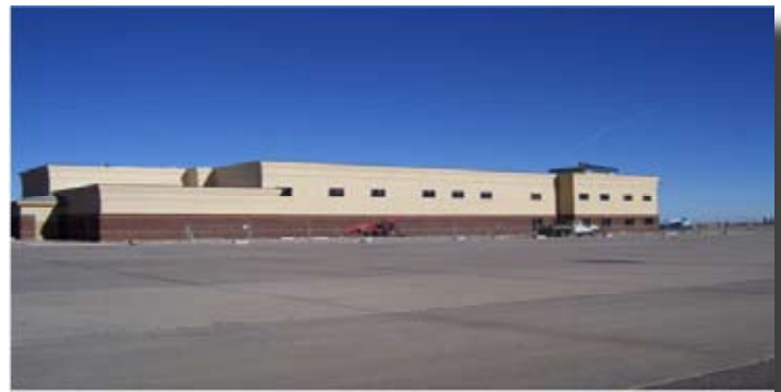
West side Squadron Operations Facility, 75% complete
