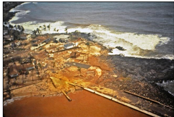
Storm Surge Damaged Homes (Iniki)
