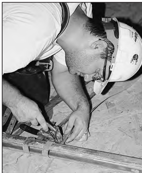
Journeyman Joey Hunt presets hangars for the commissary's air ducts.
