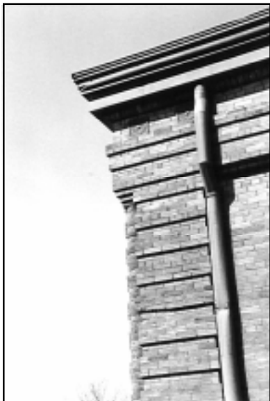
Figure 85. Drainage Pumping Station No. 1. View of upper portion of east facade of building, showing pilasters, wall, and entablature, quarter-round bricks at transition to cornice, and decorative cast-metal false key-stone on window.
