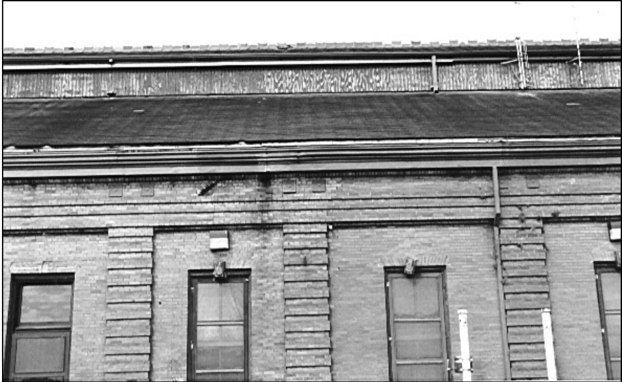
Figure 88. Drainage Pumping Station No. 1. View of roof on eastern side of building, showing decorative terra-cotta crest on monitor. The joint between the 1899-1904 masonry and 1915 construction is visible above the central pilaster.
