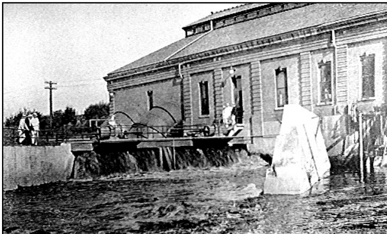
Figure 27. Testing of one 12' Wood screw pump at Drainage Pumping Station No. 1, ca. 1915. Original caption states: "...view of the discharge end of Pumping Station No. 1... pumping water from area served by Napoleon Avenue, Third Street, and Melpomene Street Canal into the Metairie Relief Canal on its way to Pumping Station No. 6. The picture shows discharge from one Wood screw pump through partly closed swinging control gates during the test. The discharge basin of this pumping station is so arranged... as to permit the discharging of the dry weather and small storm flow into the Broad Street Canal... This station is the first station designed to carry the dry weather flow across the city on its way to Lake Borgne, and thus relieve Lake Pontchartrain from the foul water which is pumped out of the city during dry weather or at the beginning of rains (from Sewerage & Water Board 1915).
