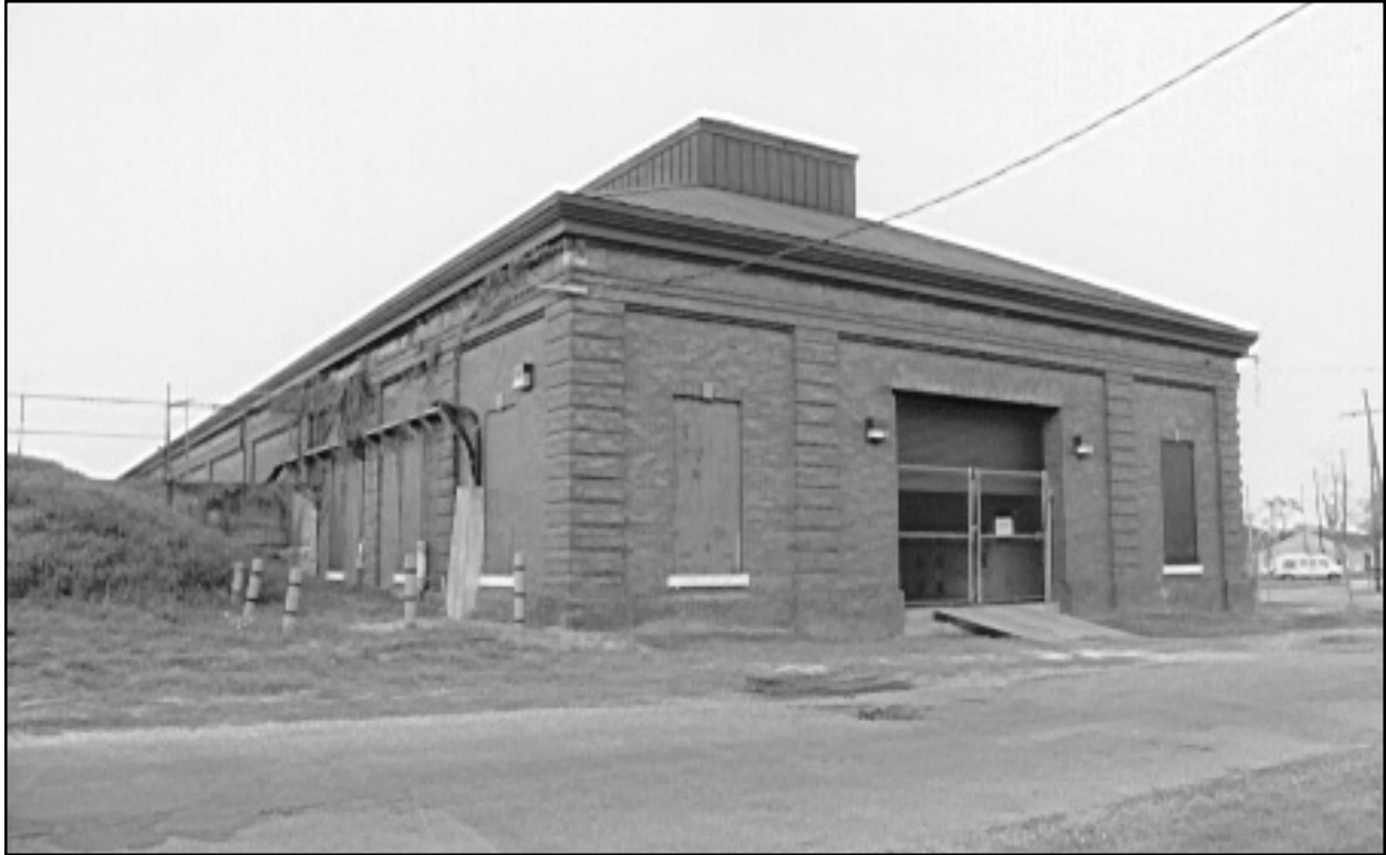
Figure 41. Drainage Pumping Station No. 3, viewed from the northwest.
