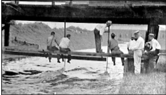
Figure 28. Testing of the 12' Wood screw pumps at Drainage Pumping Station No 1 (background), ca. 1915. Pitot tubes have been placed in the Metairie Relief Canal to measure the velocity of flow. This data was used to calculate the efficiency of the pumps. Tulane engineering students are holding the tubes while engineers record data (from Sewerage and Water Board 1915).
