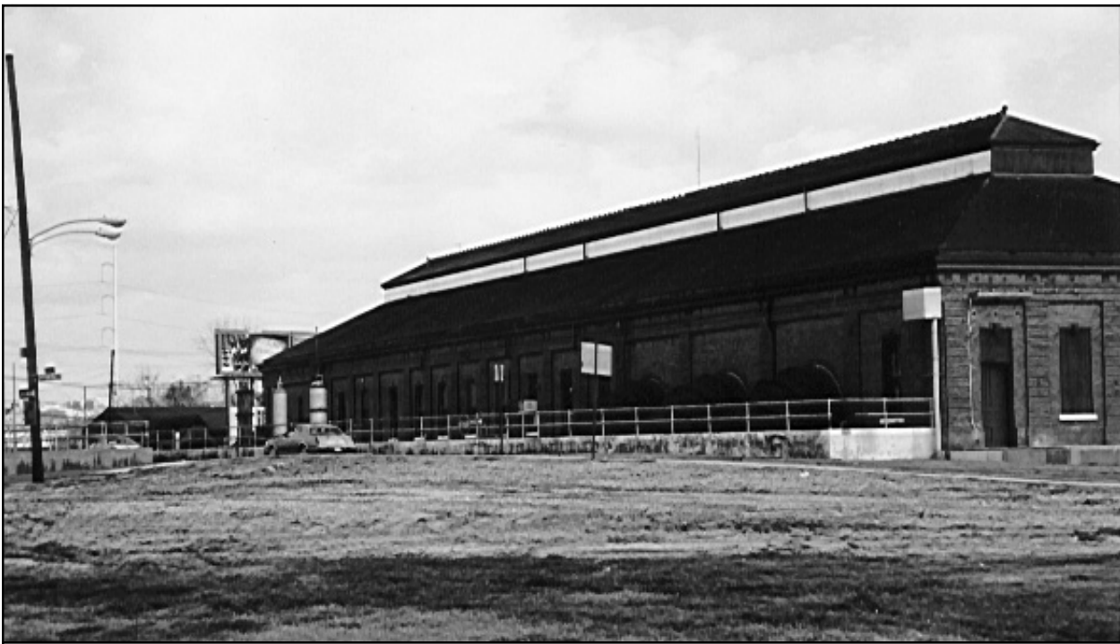
Figure 33. Drainage Pumping Station No. 1. View looking southeast.
