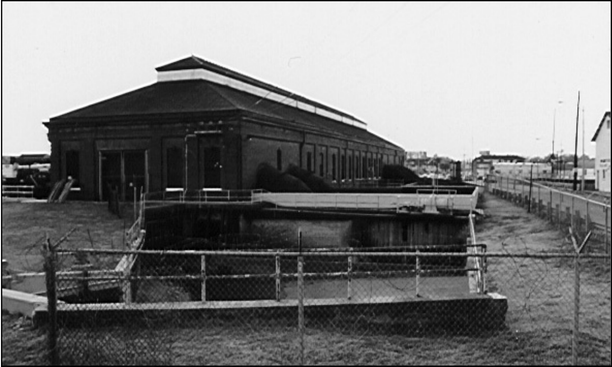
Figure 32. Drainage Pumping Station No. 1. View looking south.
