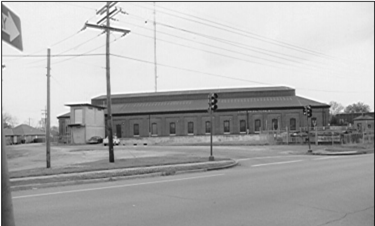
Figure 42. Drainage Pumping Station No. 3, viewed from North Broad Avenue.
