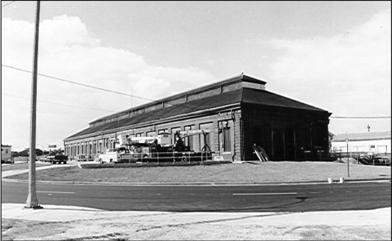
Figure 30. Drainage Pumping Station No. 1. View looking southwest.
