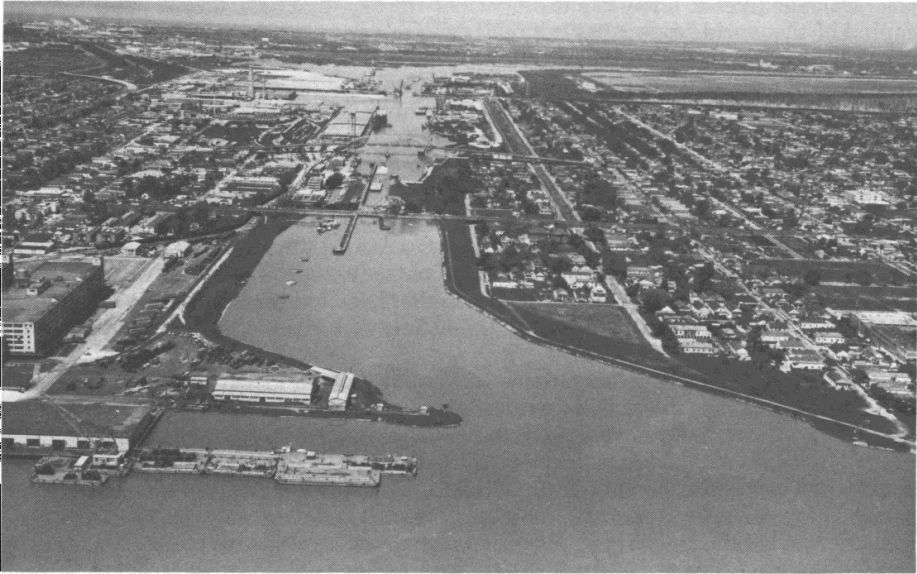
INNER HARBOR NAVIGATION LOCK AND CANAL. In use for more than half a century, the Inner Harbor Navigation Lock and Canal at New Orleans provides access to the Intracoastal Waterway and Lake Ponchartrain and is used by pleasure craft as well as large ocean-going vessels.
