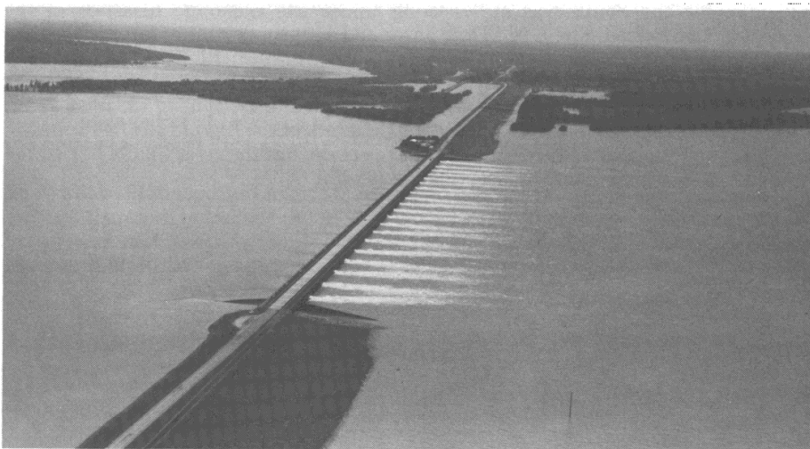
MORGANZA CONTROL STRUCTURE. During the major flood of 1973, the Morganza control structure and floodway were put in use for the first time. In the above photograph, taken during the flood emergency, the Lower Mississippi is on the left, and the floodway is on the right.
