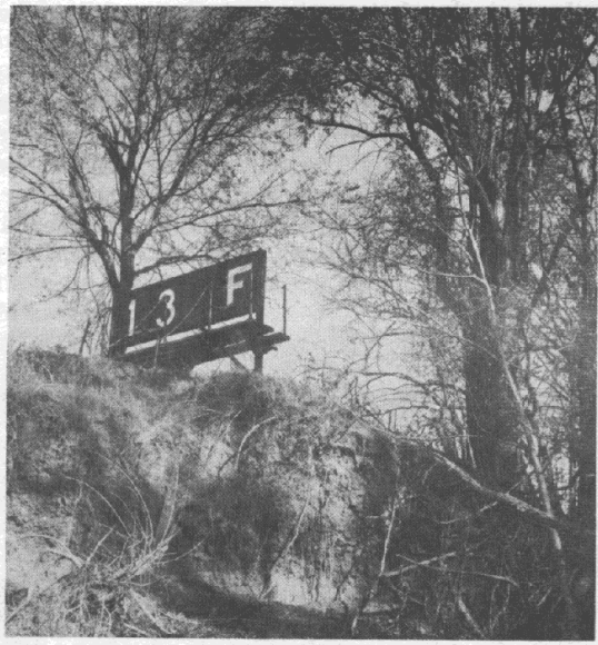
RIVER BULLETIN BOARD. Bulletin boards along the river banks keep navigators informed about stages of the water. They are maintained by the Corps of Engineers, and may seem to be an anachronism in the electronic age, when most boats are equipped with fathometers, radar, and radio communications systems, but river pilots still find them useful. When the Corps proposed tentatively that the bulletin boards be abolished, pilots protested vigorously, so the Corps continues to maintain them for the convenience of the towboat operators. In the photograph, a bulletin board located above Lake Providence, Louisiana, shows a river stage of "13 feet, and falling" at the time the photograph was taken.
