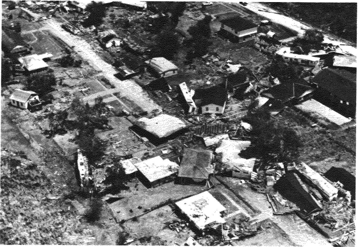
Hurricane Betsy—damage before the cleanup began.
