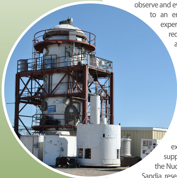
Surtsey test facility
