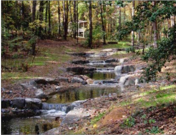
Photo 6. Step pool example (after construction).
