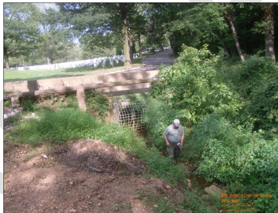
Photo 5. Looking downstream at the culvert under Ord and Weitzel Drive.
