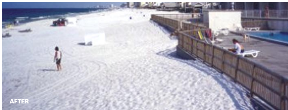
Beach nourishment, which adds sand to the coastal system, protects people and property from the effects of hurricanes and coastal storms by widening a beach and advancing the shoreline seaward. This project was constructed at Panama City Beach, Fla.
