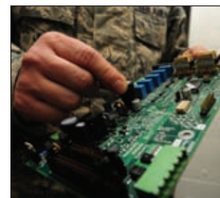
Staff Sgt. Clint Smith, 509th Civil Engineer Squadron electrical systems craftsman, checks to see if a circuit board is in operable condition, Jan. 29. Visually inspecting circuit boards for defects and damage is part of the routine maintenance electricians perform on electrical systems every day.
