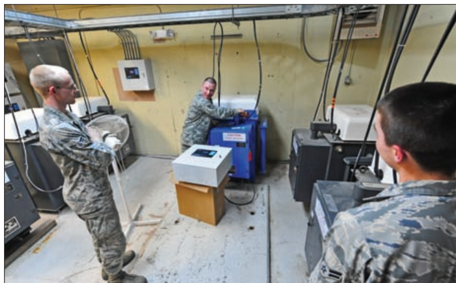
Staff Sgt. Clint Smith, 509th Civil Engineer Squadron electrical systems craftsman, trains Airman 1st Class Henry Fox, and Airman 1st Class Devin Laird, both 509th CES electrical systems apprentices, on maintaining oil filled regulators, Jan. 29. The regulators provide electrical power to various electrical systems on the flightline.
