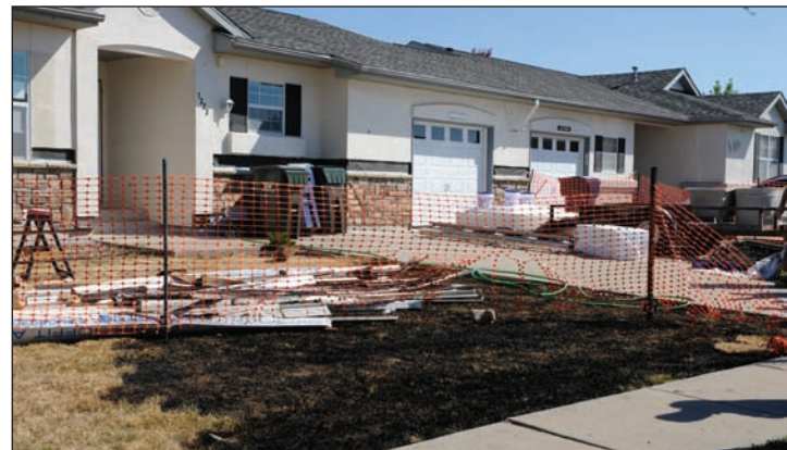
Courtesy photo A fire started July 28 in base housing, putting more than 850 Team Whiteman homes and families at risk. The 509th Civil Engineer Squadron reminds everyone to be cautious, and remain alert and aware of their responsibility to prevent fires.
