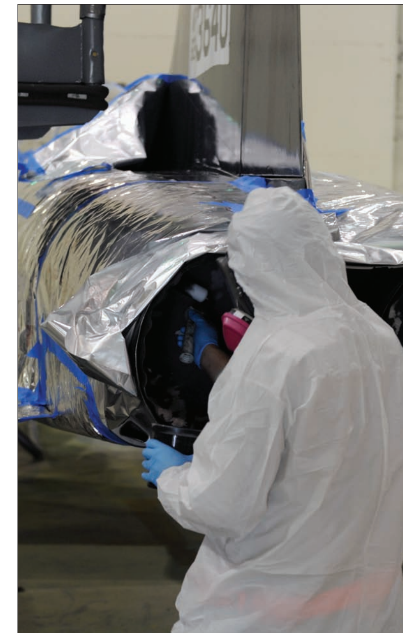
Staff Sgt. Bryan Lackey, 509th Maintenance Squadron Low Observable technician, paints the back of the T-38 Static Display during its scheduled maintenance and painting June 11. Static displays are checked for historical accuracy by ensuring color schemes and names match the time period set for the plane.
