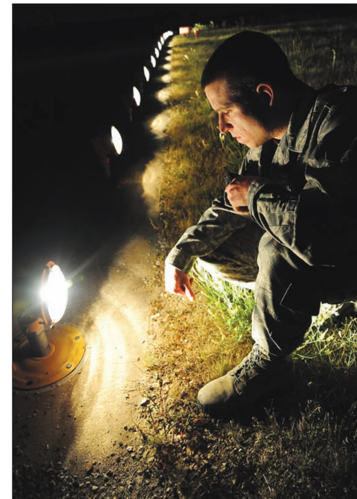
Airman 1st Class Tyler Goswick, 509th Operations Support Squadron airfield management operations coordinator, ensures runway edge lights are operational during a routine inspection June 30.
