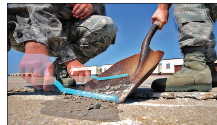
Airmen from the 509th Operations Support Squadron airfield management operations flight sweep up pieces of loose pavement from the airfield June 29, as part of an inspection for items that could cause foreign object damage.
