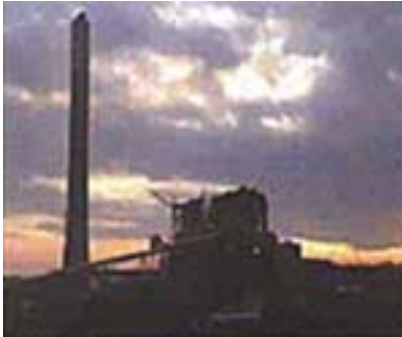
NETL's 1000-MW Rihand Power Plant, India
