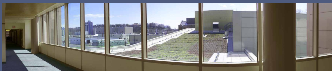
The living roof, seen here from the top floor, reduces the building's heating and cooling demands.
