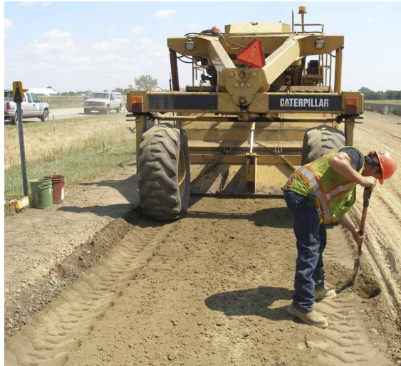
High-carbon fly ash stabilizes reclaimed pavement materials used for roadbed preparation.
